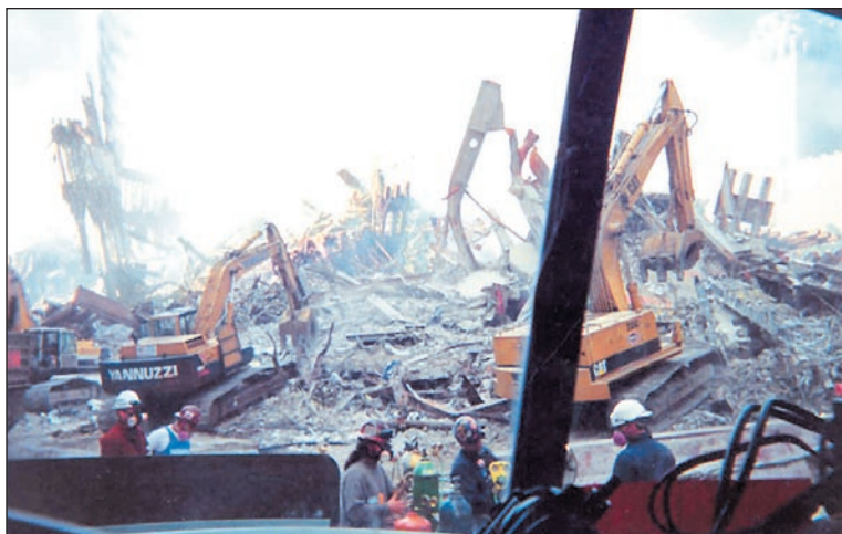
Equipment Operators Remove Debris From a Mountain of Rubble.
